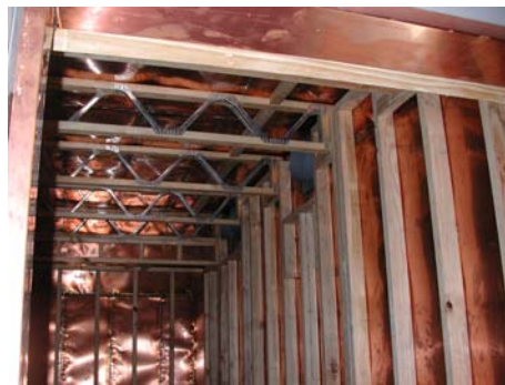
Figure 1. Framing inside the copper cladding
